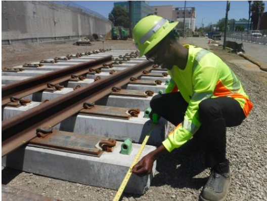
Mobolaji measures tie spacing within a BART turnout assembly.
